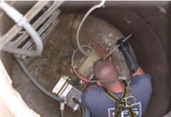
Before AAT, Mid-West Environmental's Technician performs routine internal manhole inspection.
